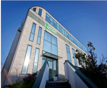
Enerdoor/Finmotor headquarters Milan, Italy
